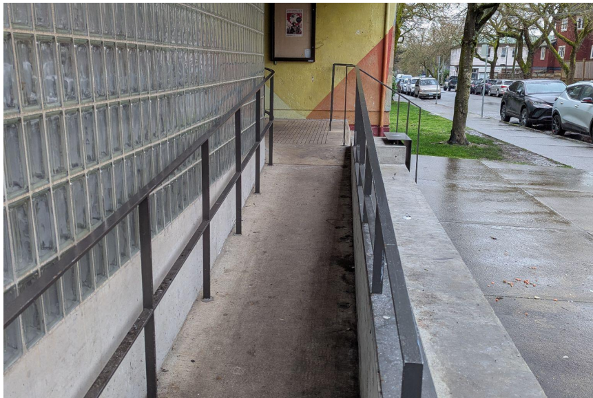
This is a picture of the ramp.
