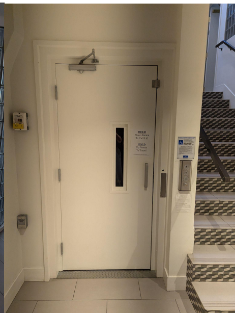
This is where the elevator comes out on the lower level.
