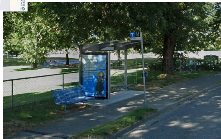
This is what the bus stop looks like on the southern side on Prior St.
